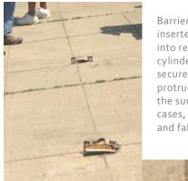
Barrier posts inserted and locked into receiver cylinders, and secured in concrete, protrude from above the surface in some cases, creating trip and fall hazards.
