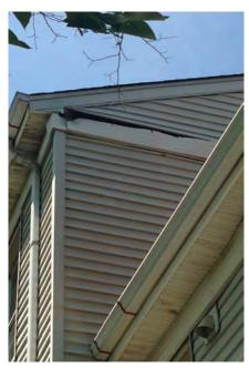
Horizontal flashing forms inverted "troughs" at the bottom of siding, which is stuffed with wiring and cables. Other cables are draped across building exteriors. Birds roost in this area, leaving droppings on the buildings and the ground, creating health hazards for residents. Siding is deteriorating in areas, creating additional areas for nesting.
