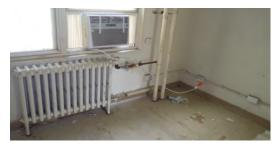
Units are heated by hot water that is piped through convectors in each room. Exposed pipes become extremely hot and have caused burn injuries. Window A/C units supplied by residents frequently overload electrical circuits and add to the condensation and mold problems in units. Some wiring is in surface mounted conduit.
