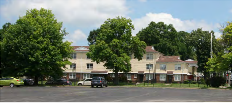
Beecher Terrace units are two and three story brick/block buildings. Vinyl siding was later added to upper floors.
