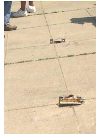
Barrier posts inserted and locked into receiver cylinders, and secured in concrete, protrude from above the surface in some cases, creating trip and fall hazards.
