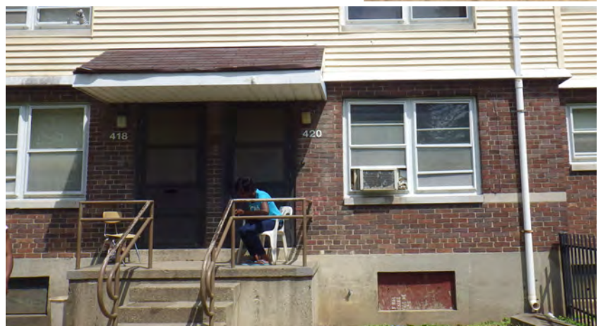
None of Beecher Terrace's units meet current ADA requirements in respect to accessibility, visitability, adaptability and visual/hearing impairment. Most units have 3 to 5 risers to the entrance.
