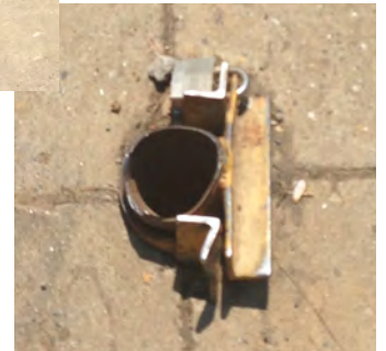
Barrier posts inserted and locked into receiver cylinders, and secured in concrete, protrude from above the surface in some cases, creating trip and fall hazards.
